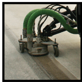
CURING COMPOUND REMOVAL
