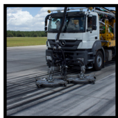
RUNWAY RUBBER REMOVAL
