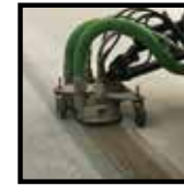
CURING COMPOUND REMOVAL
