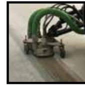
CURING COMPOUND REMOVAL
