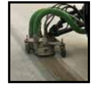
CURING COMPOUND REMOVAL
