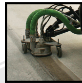
CURING COMPOUND REMOVAL
