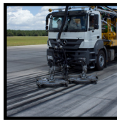
RUNWAY RUBBER REMOVAL
