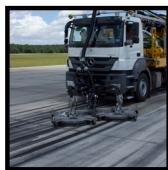
RUNWAY RUBBER REMOVAL
