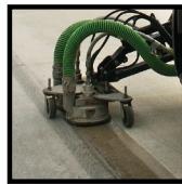
CURING COMPOUND REMOVAL
