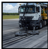
RUNWAY RUBBER REMOVAL
