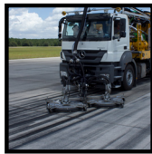
RUNWAY RUBBER REMOVAL
