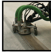
CURING COMPOUND REMOVAL
