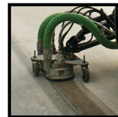
CURING COMPOUND REMOVAL
