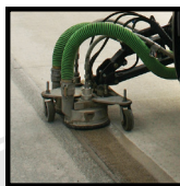
CURING COMPOUND REMOVAL
