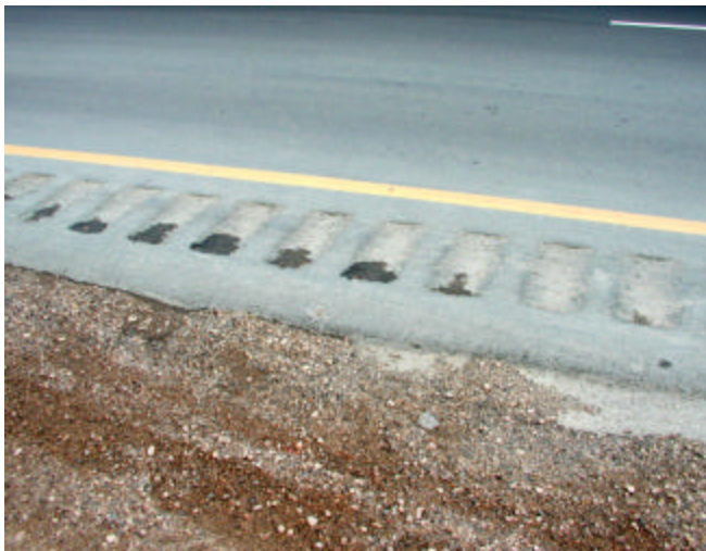
Figure 1-7: Milled Rumble Strip
