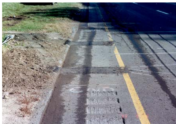
Figure 6. Rumble Strips Interrupted by Loop Detectors.
